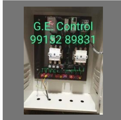
Star Delta Starter Control Panel
